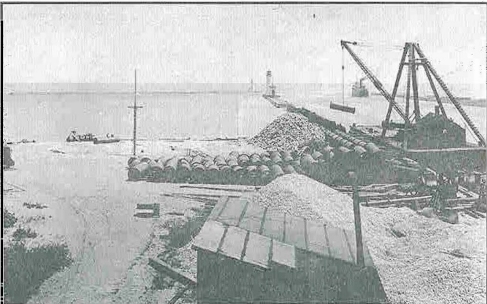
Installation of 42" Cast Iron Intake Pipe into Lake Michigan - 1916
