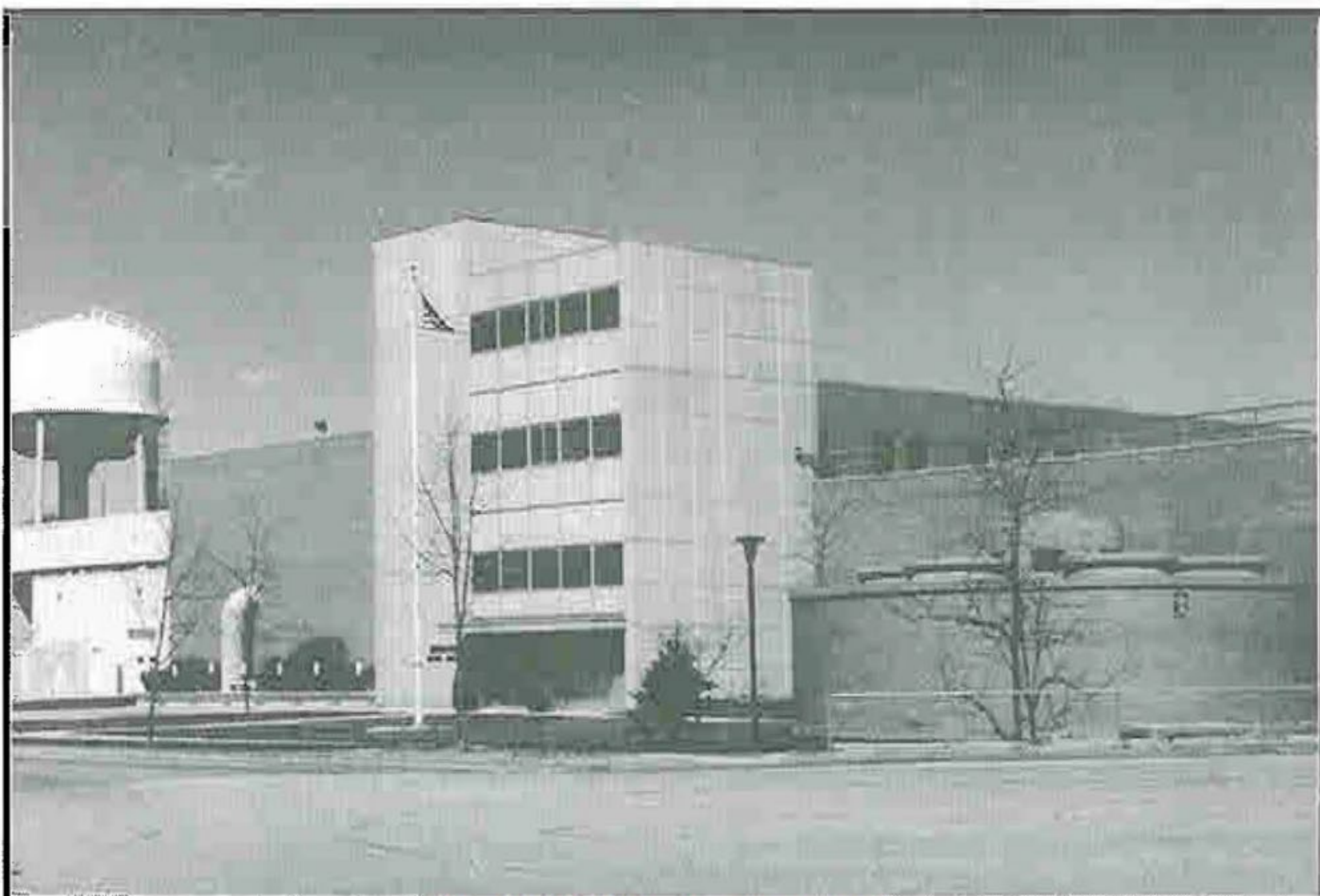
New 20 MGD Filtration Plant - 1964
