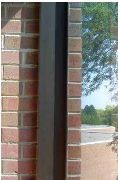
Brick exteriors and interiors, separated only by glazing with no applied finishes.
