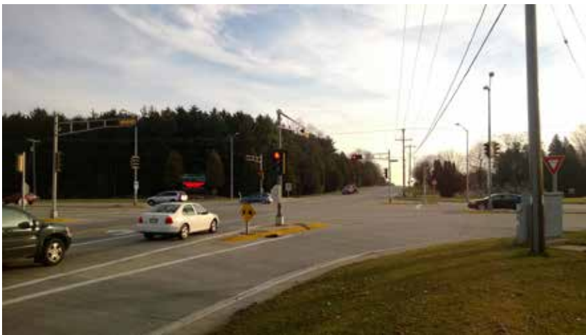
The existing campus identity signage at Green Bay Road and CTH E is scaled for motorists.
