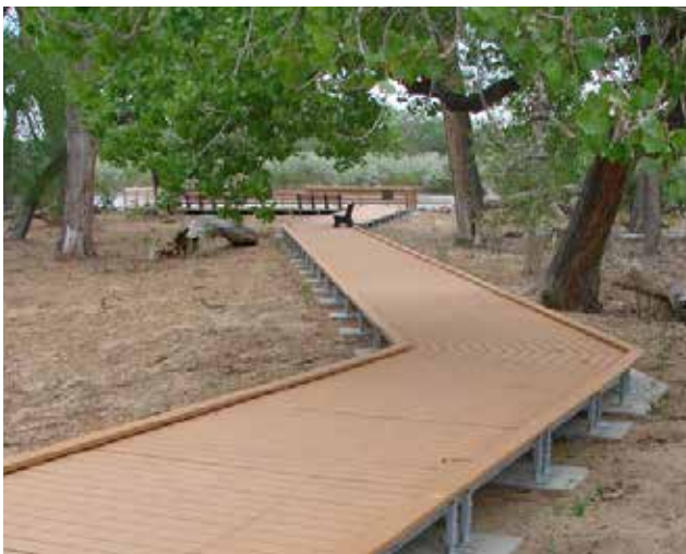
Boardwalk with plate connections
