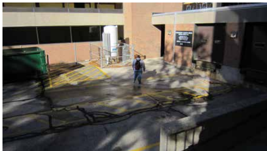
The Greenquist loading dock area is often used for pedestrian circulation.
