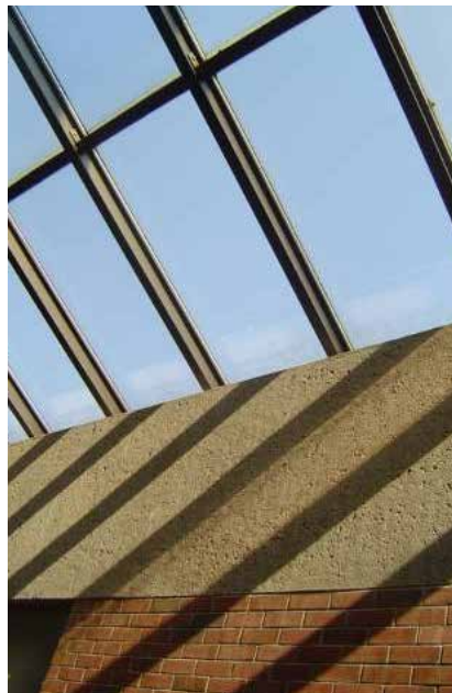
Skylights, exposed concrete and brick combine to create colorful and patterned walls.
