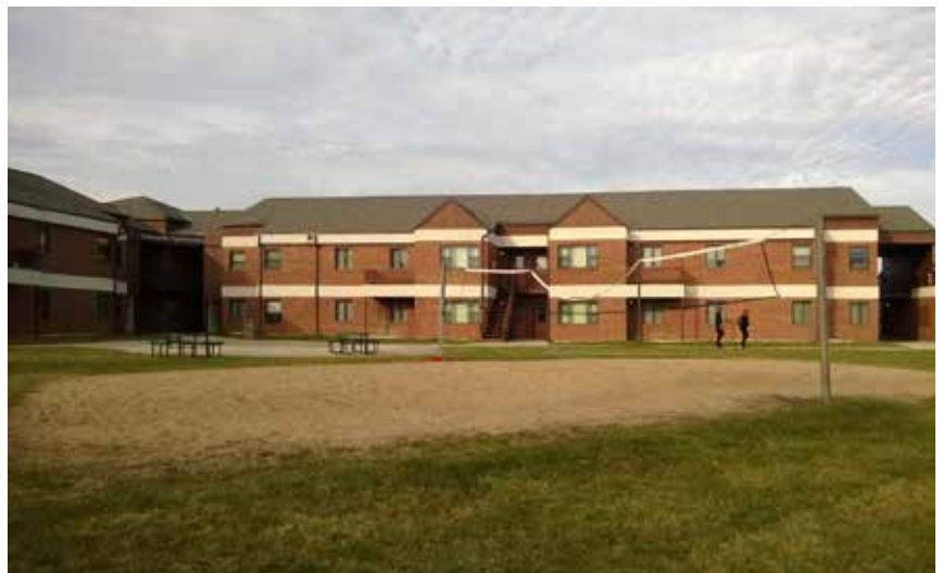
With recent roof and membrane investments, University Apartments will serve the university for another decade.
