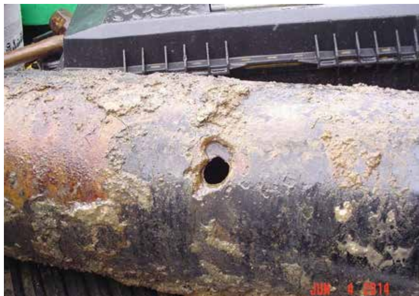
A recently excavated ductile iron pipe has evidence of severe corrosion.
